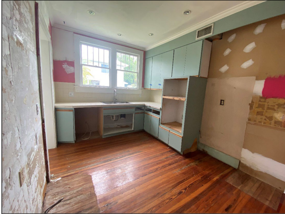
Figure 3: Kitchen prior to rehabilitation
