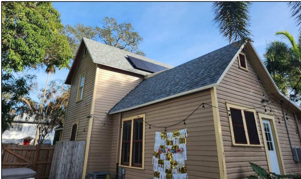
Figure 2: North (side) and west (rear) elevations of subject property.
