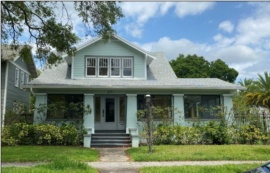
Figure 1: Front façade of subject property, with enclosed porch
