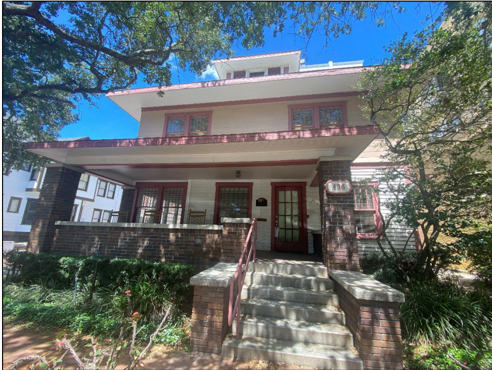
Figure 1: Front façade of subject property
