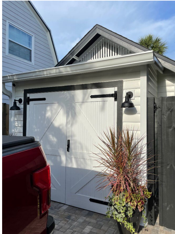
Figure 5: New front façade with reconstructed carriage doors.
